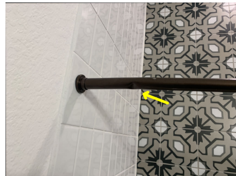
Damage/dent observed on the shower curtain rail; Level 1 Room 1
