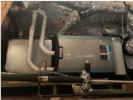
Furnace-1 located in the Attic
