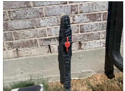
Water Shut off valve located on west side of building
