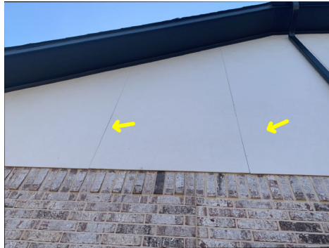
Observed opening/unfinished exterior wall on both (west/east) sides of the building
