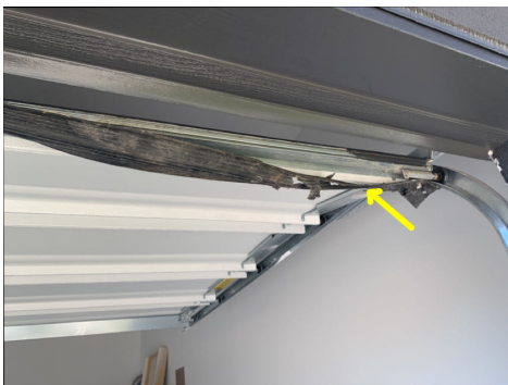
Main entry garage door weather-stripping damaged
