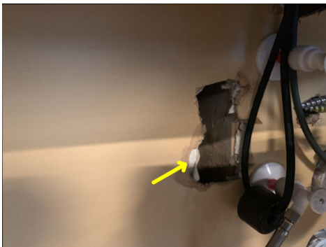
Wall opening under kitchen cabinet require repair
