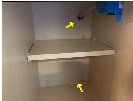
Opening and incomplete finishing; kitchen cabinet
