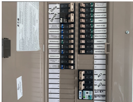
Electrical panel breakers properly identified
