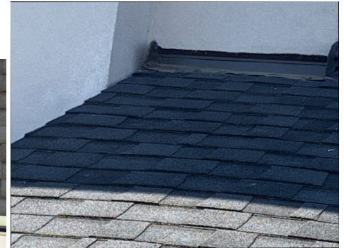
Flashings checked at the penetration
