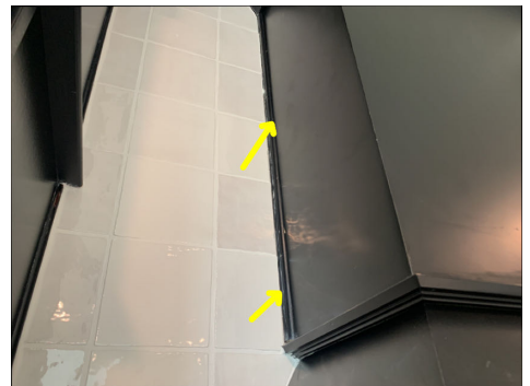
Caulking required to seal openings on both sides of the Range Hood
