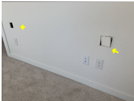
Wall openings require repair; level 2 - Bedroom 1
