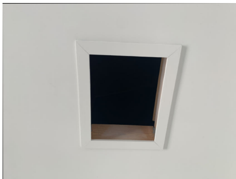
Missing hole cover in main garage
