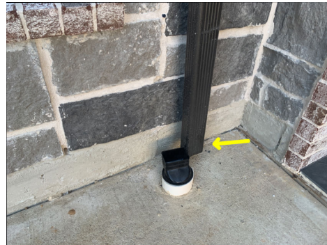
Incomplete downspout installation
