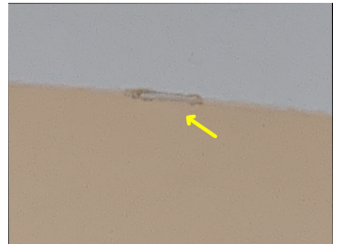
Wall damage on front arch decking require repair
