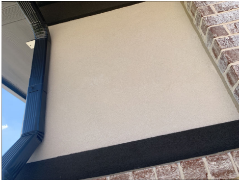
Stucco finishing on exterior wall
