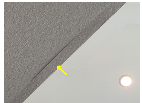
Tape revealing require repair; living room/kitchen ceiling area
