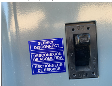
200 Amps service disconnect located on the west exterior wall
