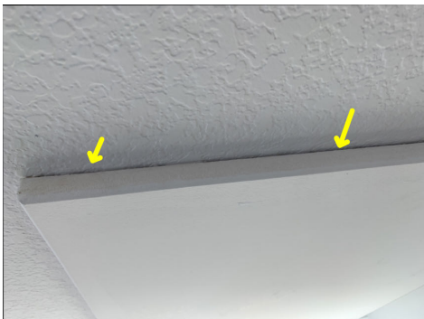
Caulking required to seal openings; Theater room
