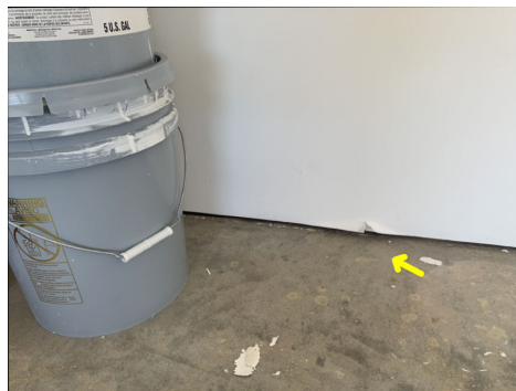
Opening in main garage floor require repair
