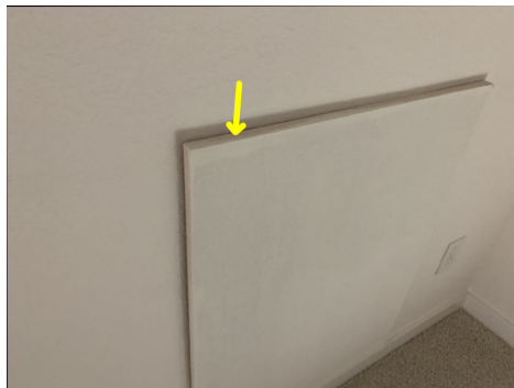
Caulking required to seal openings; Level 2 Room 1
