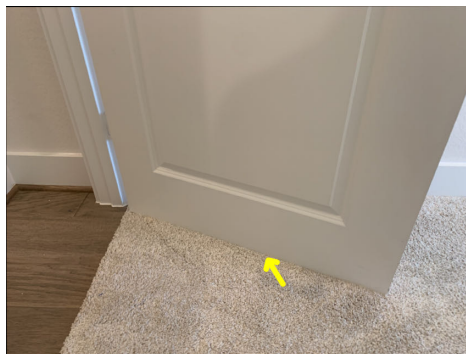
Entry door stuck and unable to open; Level 1 Bedroom 1
