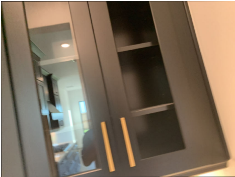
Glass covering on storage cabinet missing; Kitchen area
